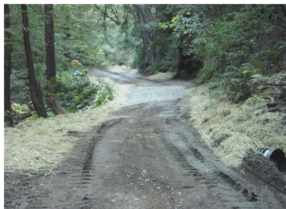
Figure 7-4 Exposed soil has been mulched
