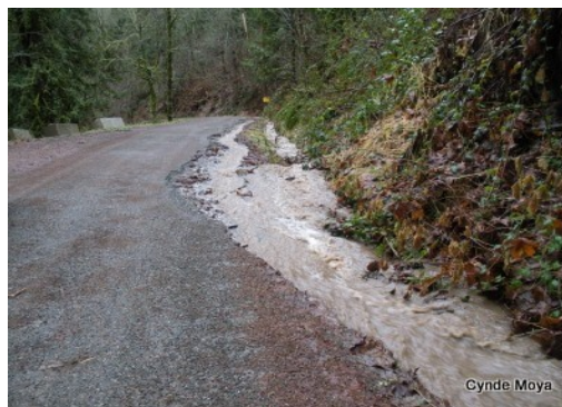
Figure 7-19 The result of an undersized/clogged ditch
