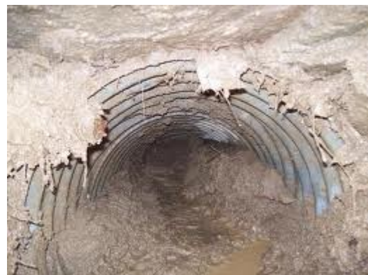
Figure 7-24 Culvert clogged with sedi-
