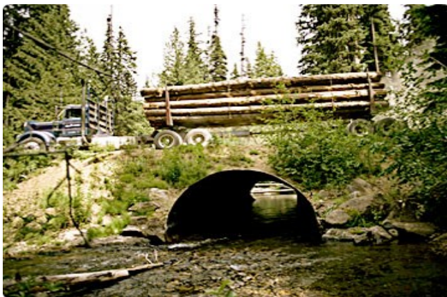
Figure 7-20 Fish friendly arch culvert over low grade stream
