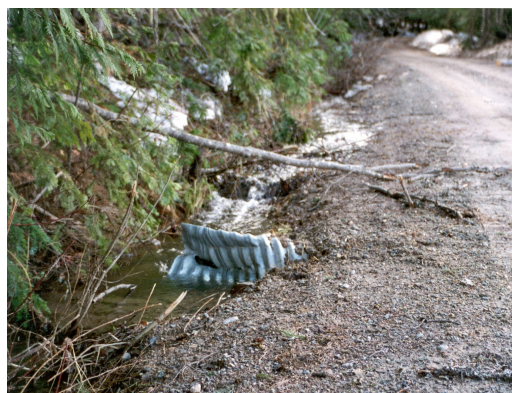
Figure 7-6 Crushed culvert cross drain
