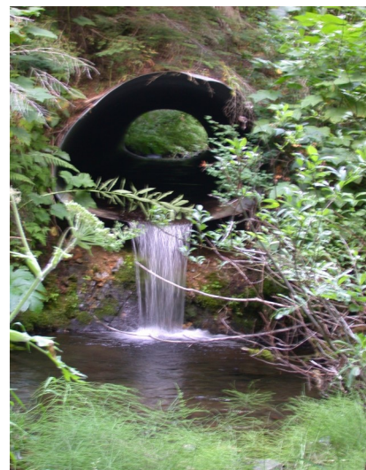
Figure 7-27 Culvert is too high, creating a vertical barrier for fish and scouring at outlet
