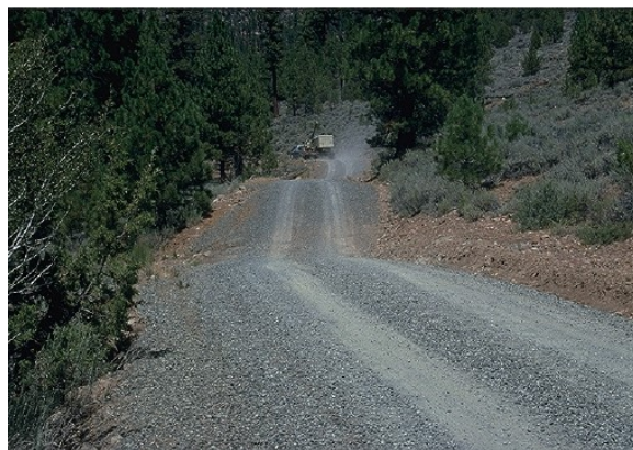
Figure 7-5 Road constructed with outward sloping rolling dips
