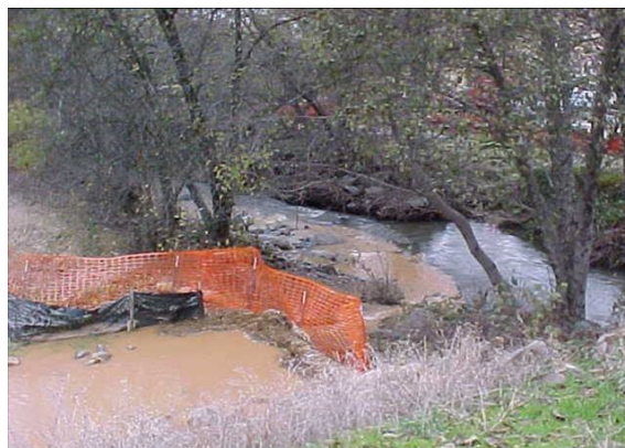
Figure 7-3 Poor placement of BMPs may result in sediments entering streams.
