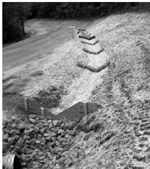
Figure 7-16 Straw/fiber wattles used as check dams in ditch to slow runoff
