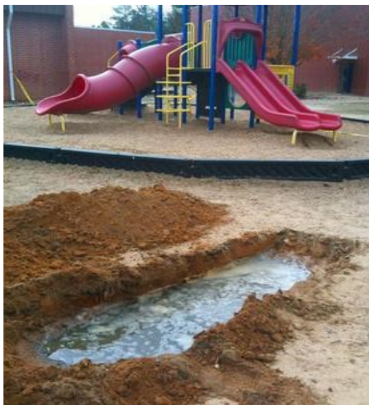
Failed septic system on playground.
